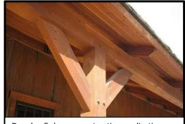
Douglas-fir beam construction applications
